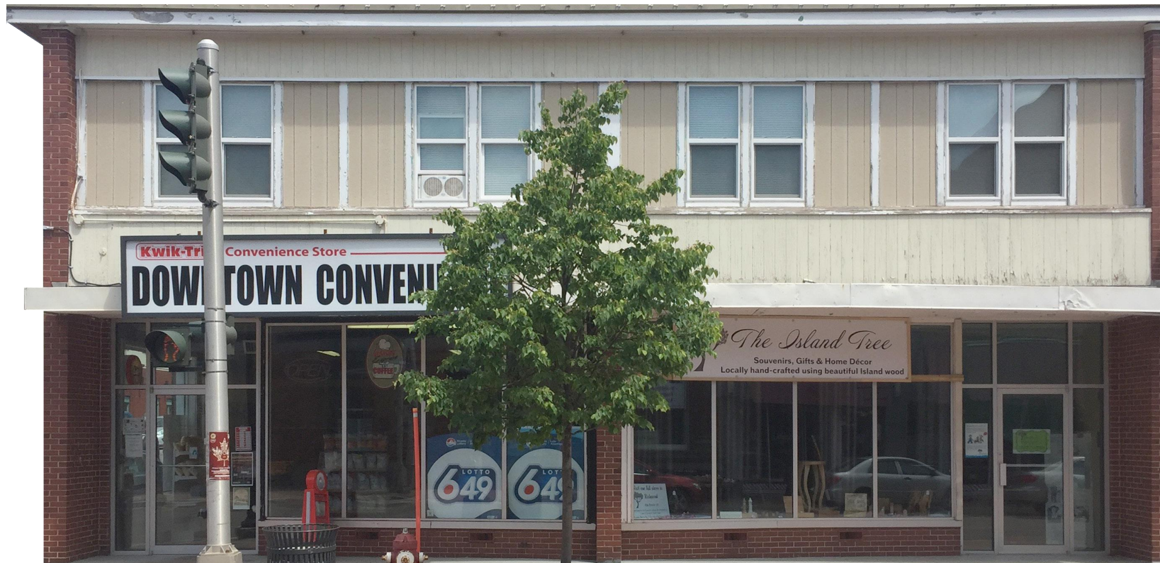
FIGURE 66. Facade Program Before
